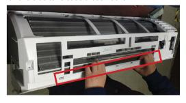
Press below position to unfasten the hooks in side of Front Panel, then take the Front Panel out.
