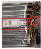
9) Remove 2 screw fixing the Ground wire.
